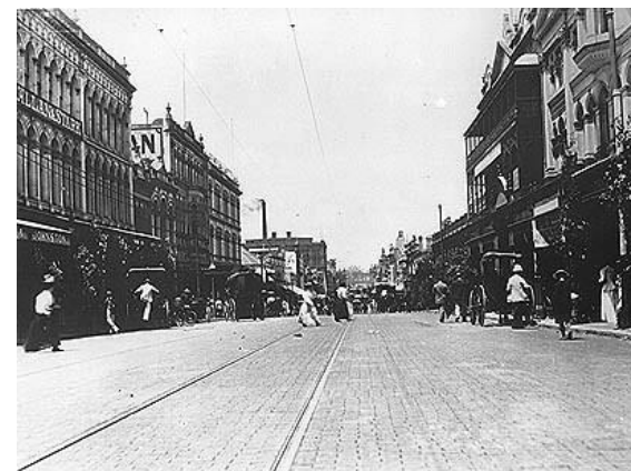
Wooden blocks laid in Queen Street, Brisbane
