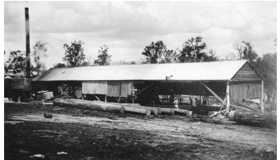
Fredin's sawmill at the One Mile Creek. Water for the steam engine to drive machinery was pumped from the creek.
